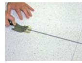
Welding bead is trimmed in two steps, with an initial trim using a trim plate.
