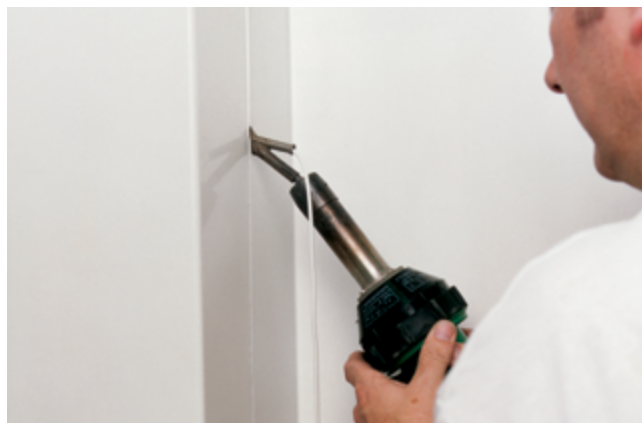
Heat welding Altro Whiterock panels together
