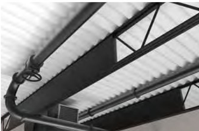
InvisAcoustics™ Panels in Black Truss Installation
