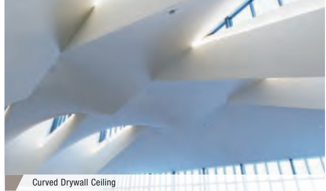
Curved Drywall Ceiling
