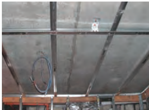
QUIKSTIX™ Drywall Grid System with Locking Pocket Main Beams
