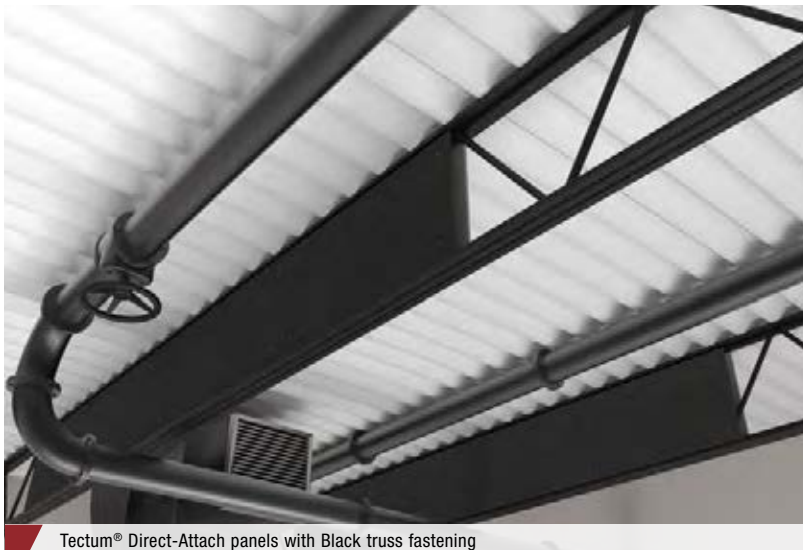
Tectum® Direct-Attach panels with Black truss fastening
