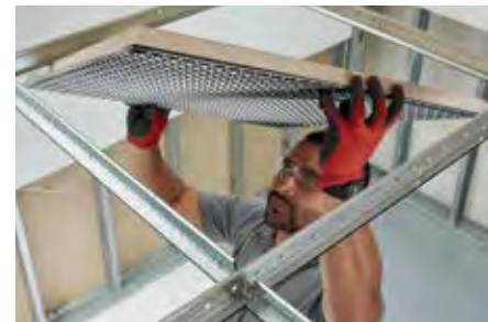
MetalWorks™ Mesh ceiling panel with Calla® 2820BK infill panel for high NRC performance
